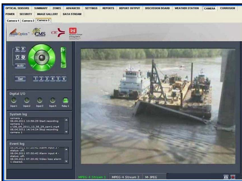
A screen grab from the SHM system depicts barge removal efforts along the I-20 Mississippi River Bridge.
